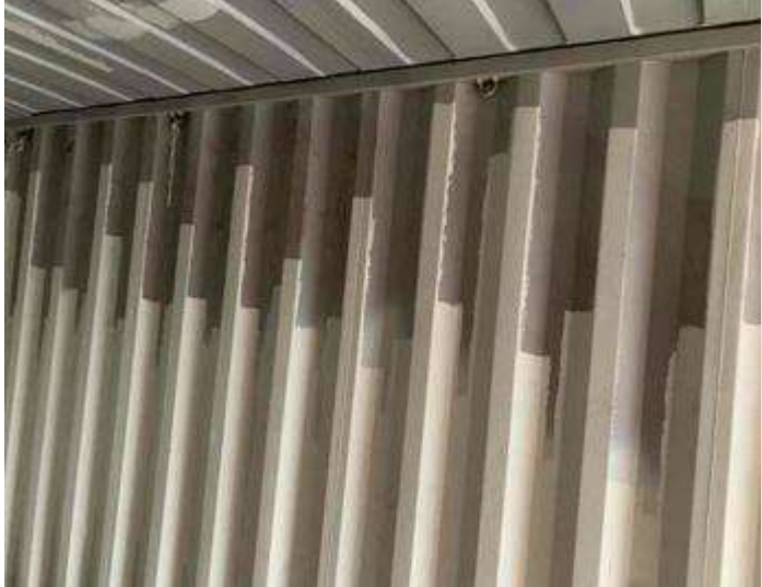
8.1.5. No defects inside container WALLS (Left & Right) 集装箱内侧墙面缺陷
